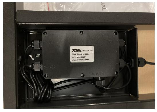
Unscrew all 6 screws in the junction box. Remove the plastic junction box lid and see if no wires are loose.
